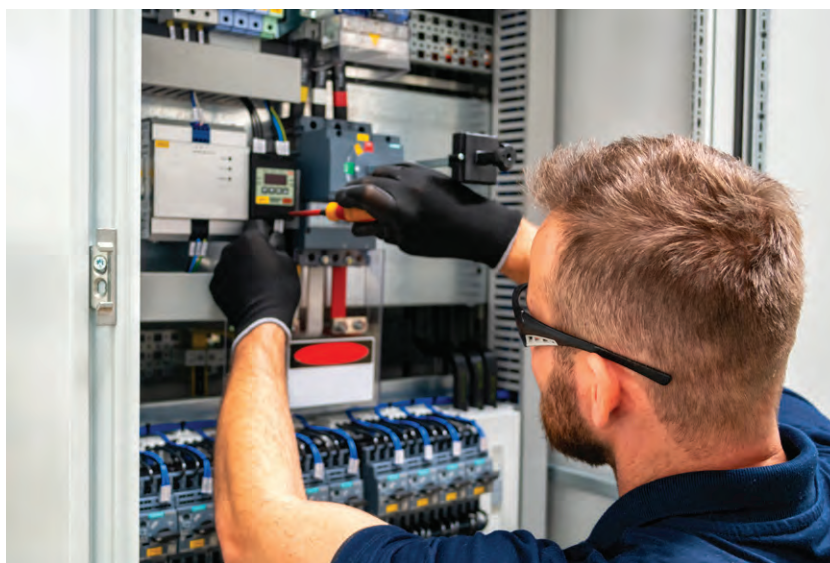
Image 10. Electricians will require hydrogen upskilling
