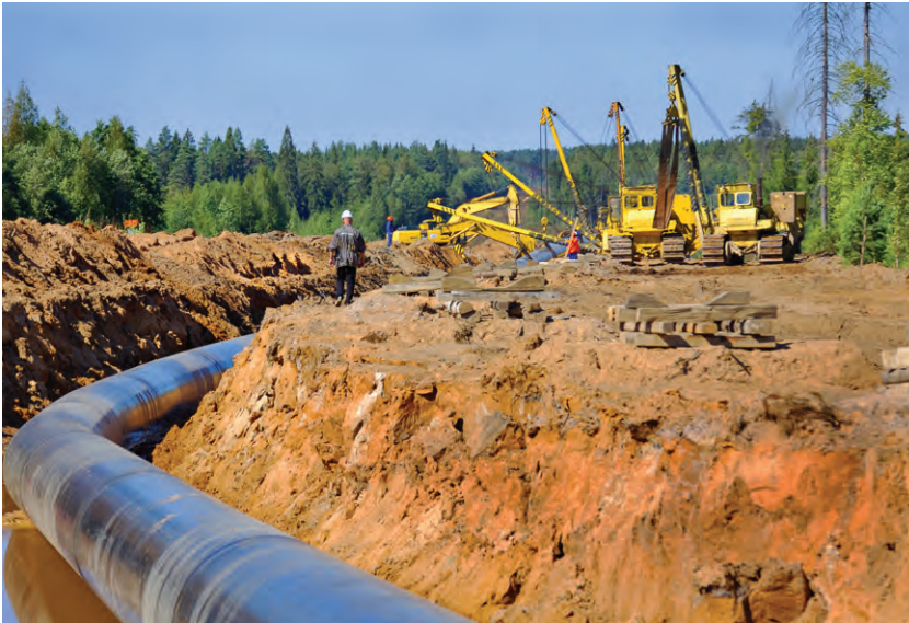
Image 7. Construction of a gas pipeline
