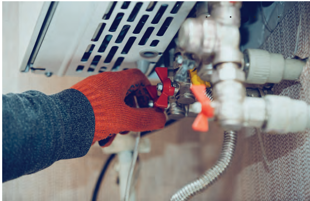
Image 9. Gas fitters ensure safe and effective connections between distribution gas pipes and appliances
